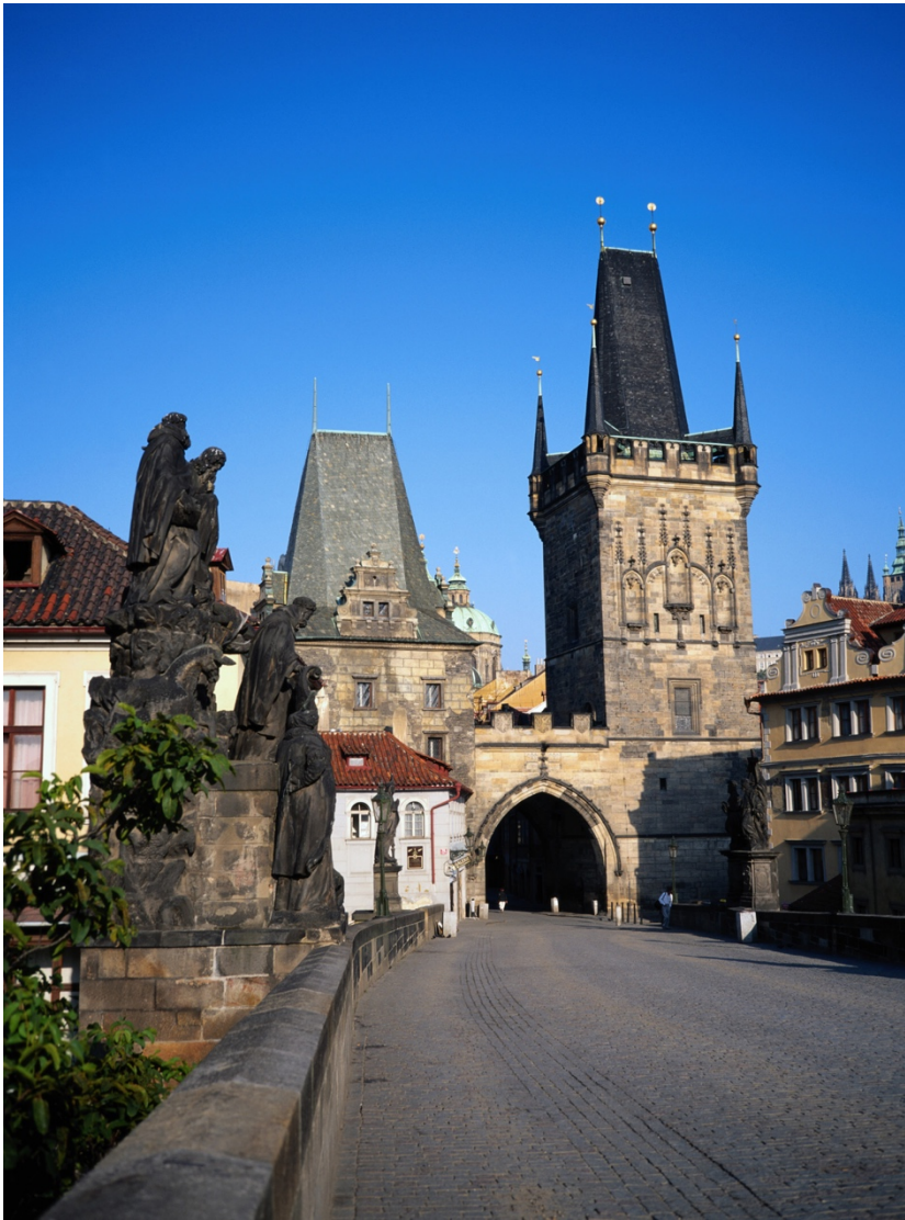
Charles Bridge - Prague
